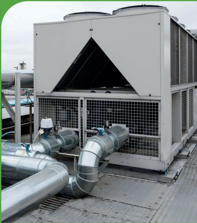
Air Cooled Chiller System
