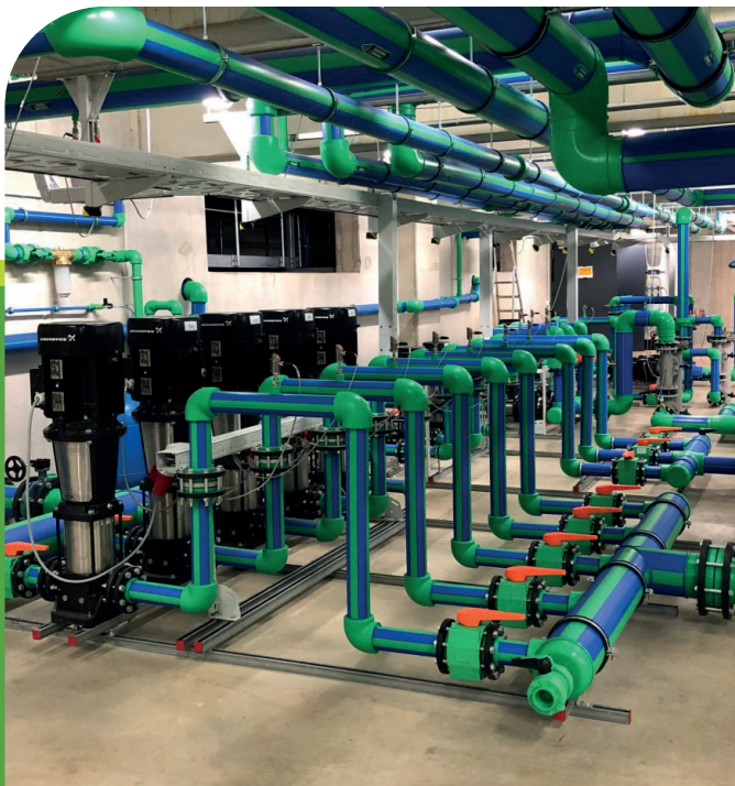
Transfer Pumps (Cold Water System)
